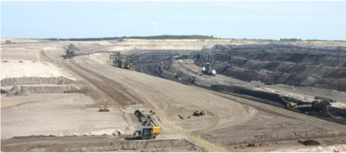
Figure 1: Excavation (in the left) and dumping (in the right) of overburden material in an open pit-lignite mine in the Lusatian mining district, Germany
